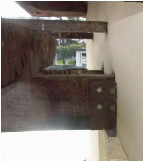
Bolts connecting north pergola to north small loggia are believed to have been added in 2004 when the trellis was rebuilt.
