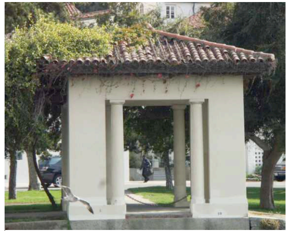
South loggia showing missing roof tiles and potential damage from vines.
