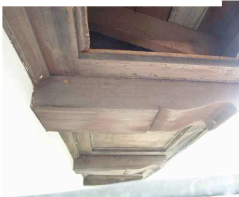
Unpainted redwood soffit in excellent condition on the North loggia.
