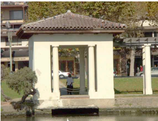
Small loggia on North side, showing missing roof tiles and stream outlet below floor.
