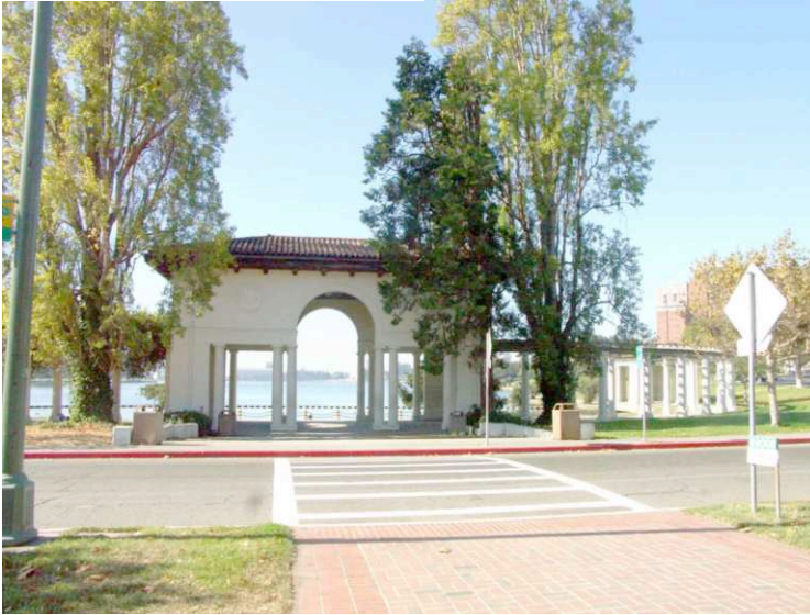
Main loggia as seen from El Embarcadero Street.
