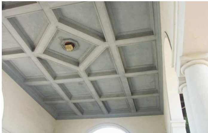
Coffered ceiling of main loggia.
