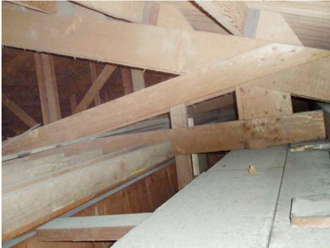
Attic of main loggia, showing sill plate bolted to concrete wall, but no shear connection between plate and roof.
