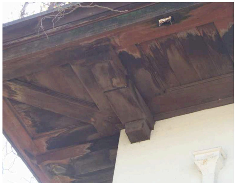
Stained soffit and missing downspout at SE corner of main loggia.
