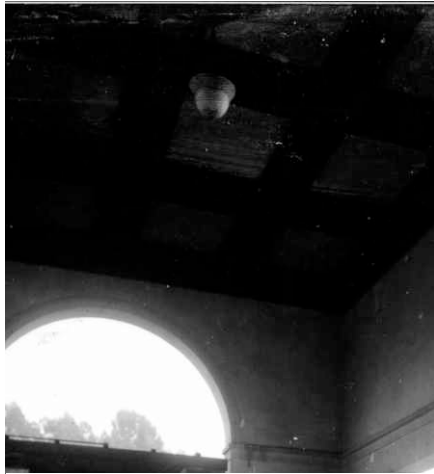
Historic light fixture is barely visible in this historic photograph of the interior of the main loggia.
