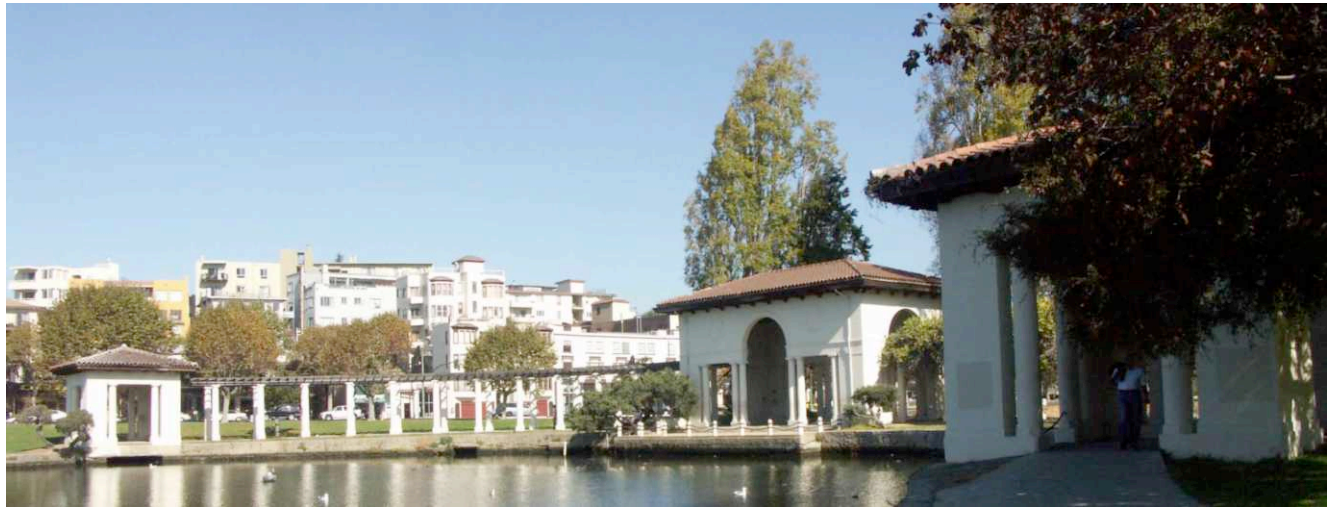
Current and historic views of structure. Main loggia is in center, South loggia is at right, north loggia across water at left. Curved pergolas join the three loggias.
