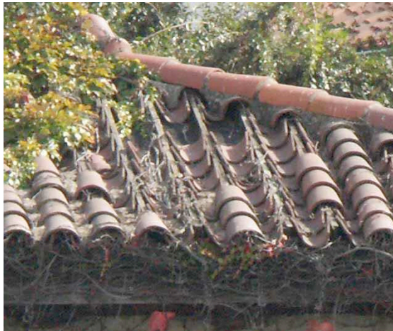
Above: approximately 50 missing cover tiles on the South loggia leave pan tiles exposed. Wood battens are visible between columns of pan tiles.
