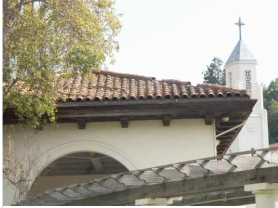
Main loggia with missing hip tiles.
