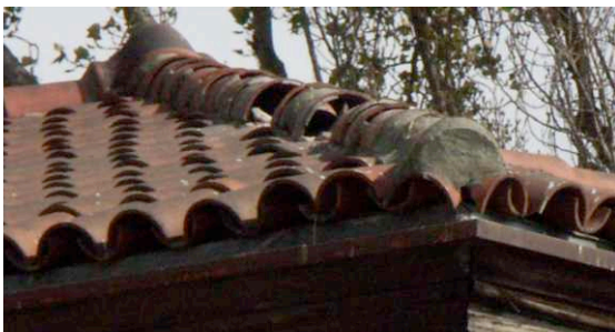
Below: ridge cover tiles and special cap tile on main loggia. Apex tile is visible at the top.
