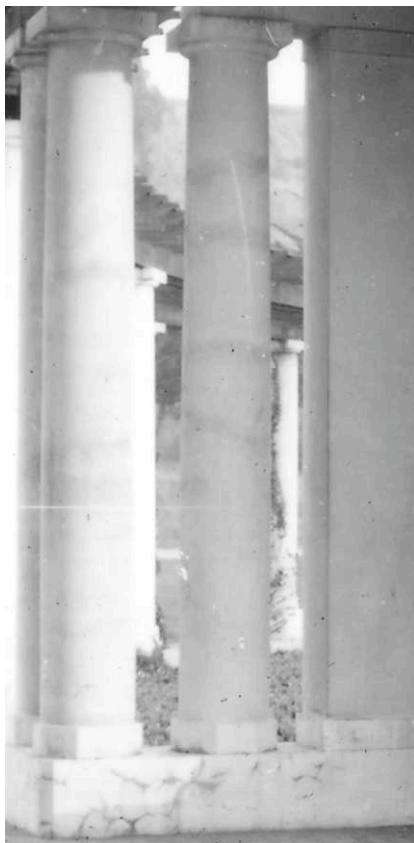
Enlargement of historic photograph, showing faux marble paint on columns and base of wall.
