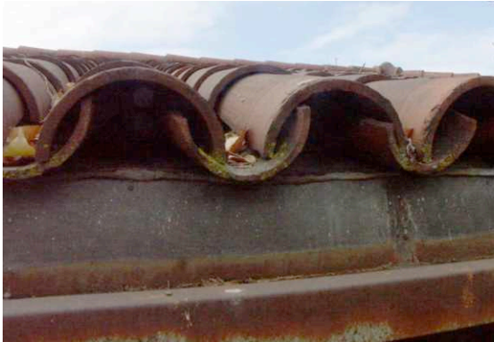
2-piece tapered mission tiles are 9 1/8" wide x 18" long. The profile is a full half circle. The wide end of the cover tiles and the narrow end of the pan tiles are visible in this photo.
